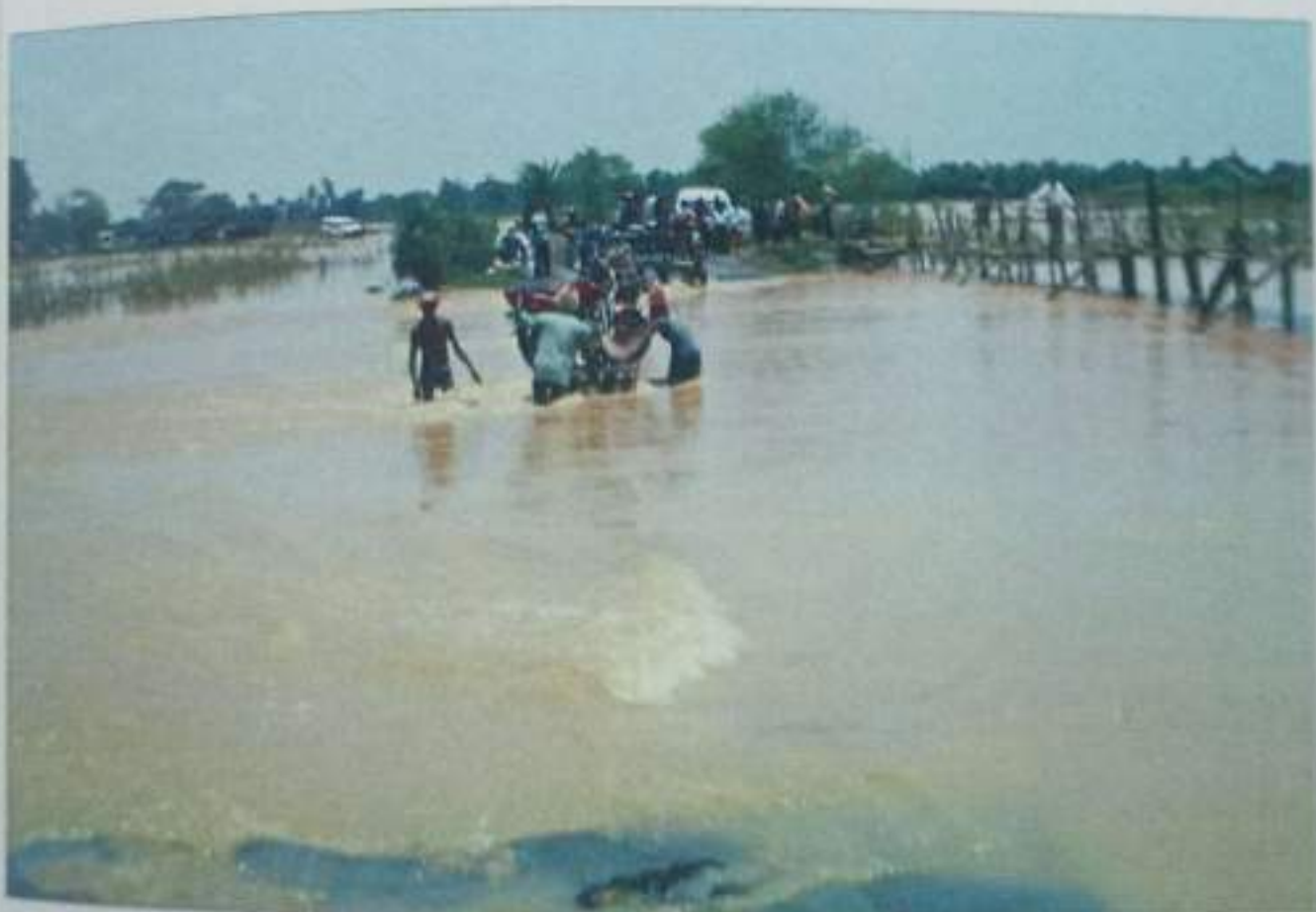
Causeway at 16km of Bhadrak-Kothar-Aradi road in Dhamnagar Block of Bhadrak District
