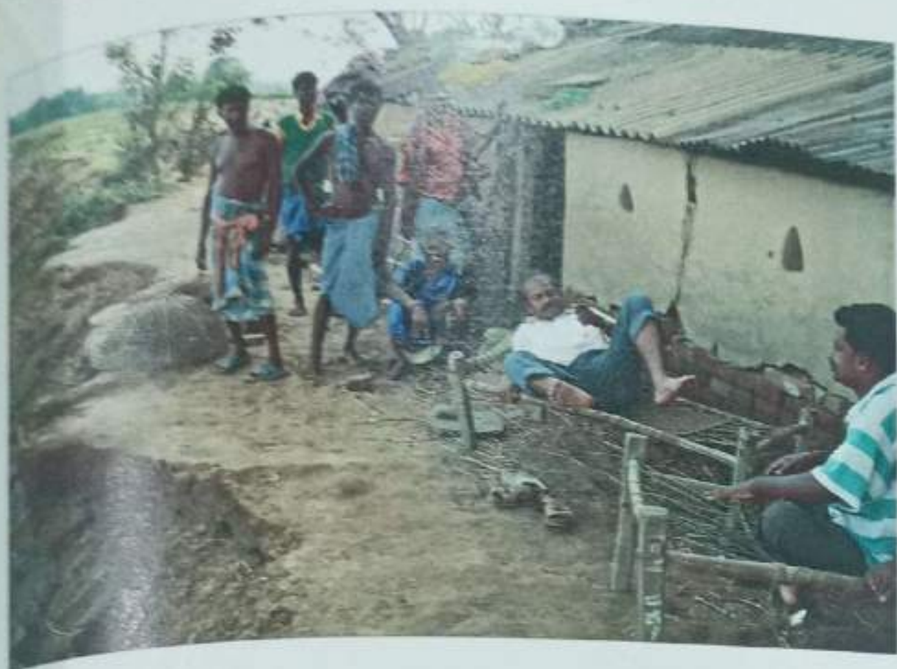
Jaleswar-Kuanrpur-bank scouring in Baleswar District
