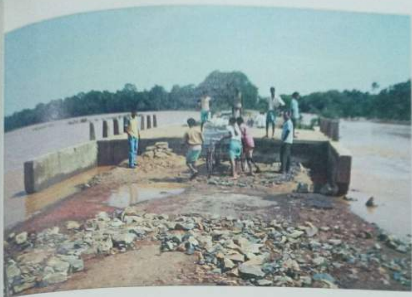
Bhadrak-Dhamnagar-Dobal-Sendhapur road 6.650 km in Bhadrak district
