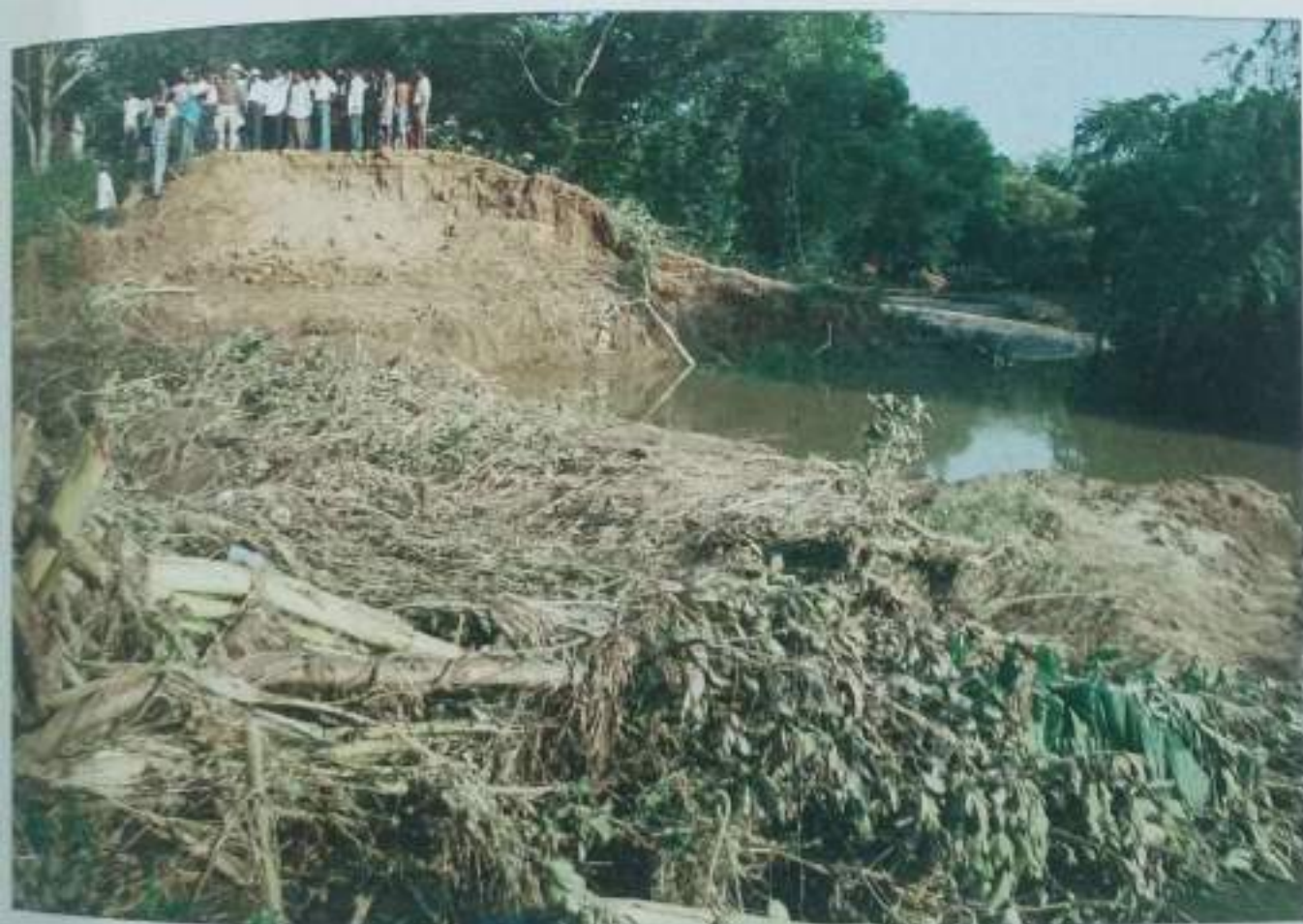
Baliapal-Palapada flood embankment in Baleswar District –Subarnarekha right
