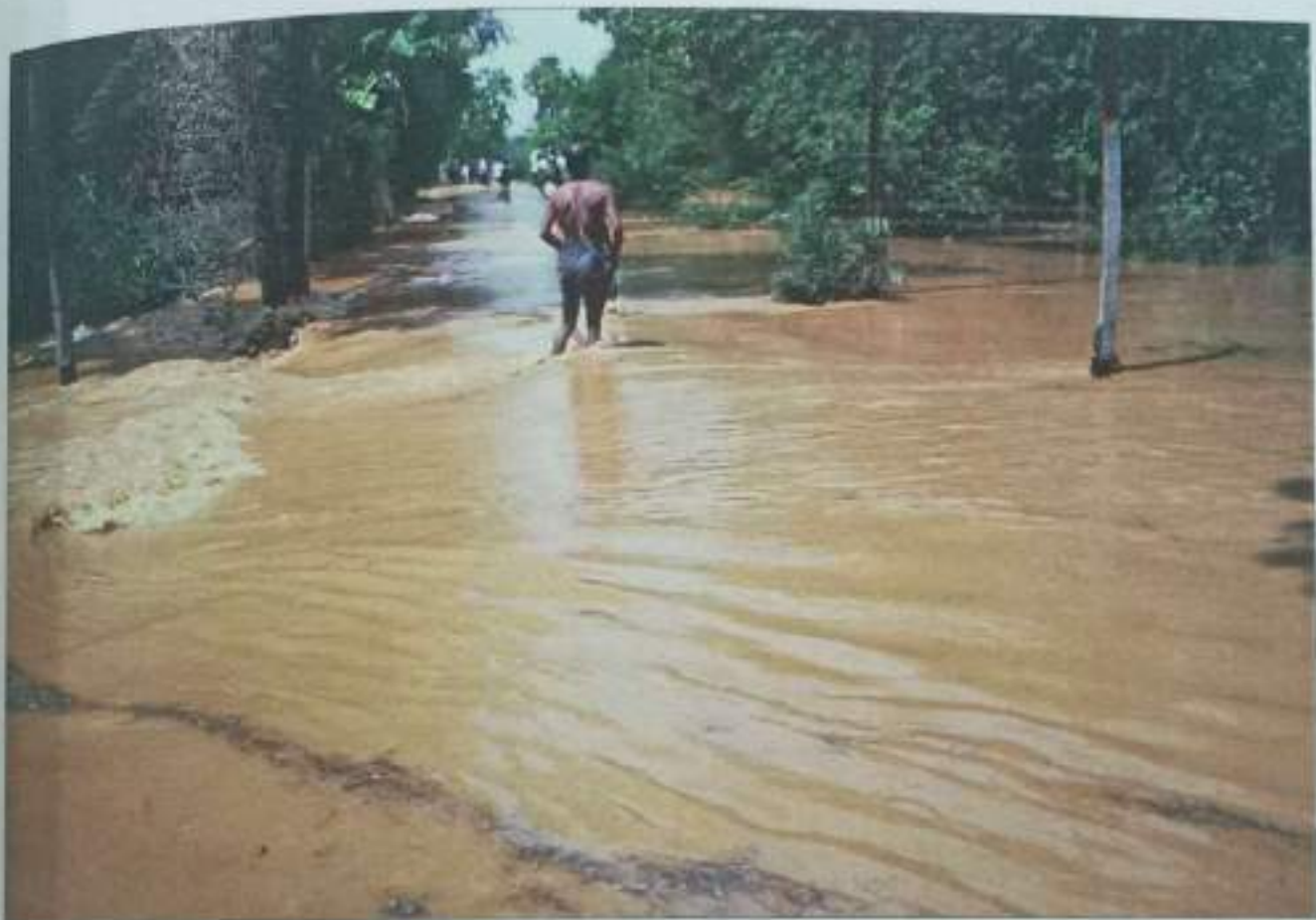
Dhamnagar-Dobhal-Sendhapur road at 2 km to 3km of Dhamnagar Block in Bhadrak District
