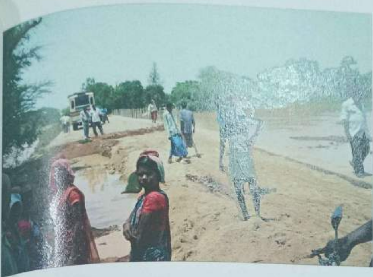
Restoration work at 3.550km of Dhamnagar-Sendhapur road in Bhadrak district
